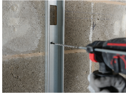
Gypframe 'C' Studs are suitably fixed to abutments.
