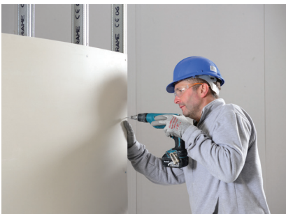
Gyproc plasterboards or Glasroc specialist boards are then fixed to the Gypframe framework with Gyproc Drywall or Jack-Point Screws. The plasterboards are fixed horizontally, with all joints staggered. Additional studs may be required where multiple layers are specified to account for the difference that arises between inner and outer radii.
