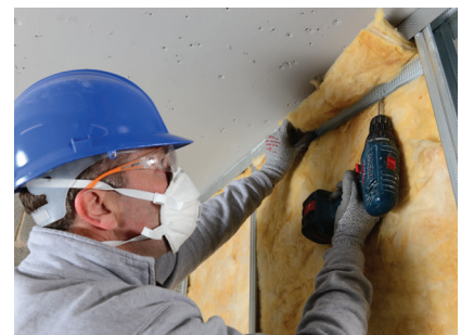
Isover Acoustic Roll insulation can also be included within the partition cavity for optimised acoustic performance.
