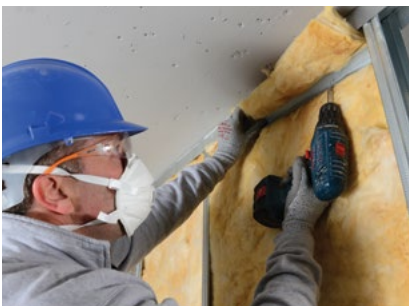
Isover acoustic insulation can also be added to the partition cavity for increased acoustic performance.
