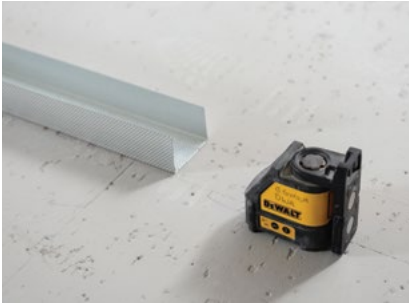
Gypframe Deep Flange or Extra Deep Flange Floor & Ceiling Channels are suitably fixed to the floor and soffit.
