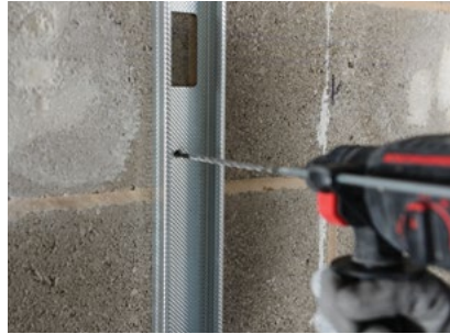
Gypframe Studs are suitably fixed to abutments.
