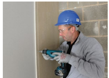
Rigidur boards are then fixed as the outer layer to all Gypframe framing members with Rigidur Screws.
