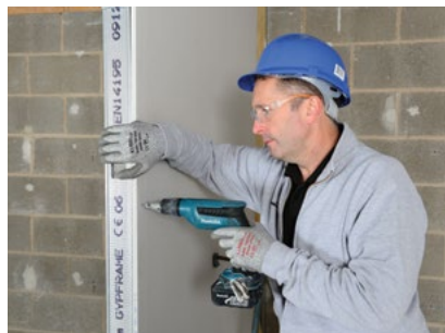
Gyproc DuraLine, Gyproc SoundBloc or Gyproc WallBoard plasterboards may be installed as an inner layer with Gyproc Drywall Screws.
