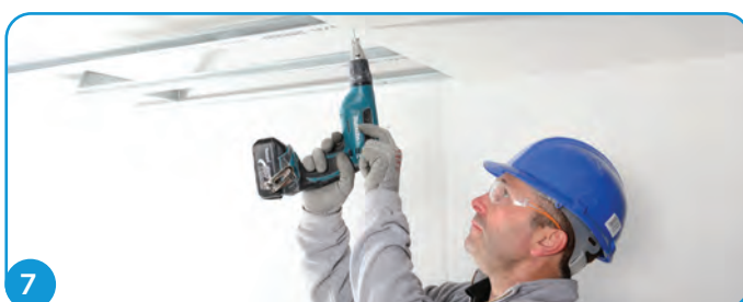
5 Position Gyframe MF7 Primary Support Channels then use Gyproc Wafer Head Jack-Point screws to fix the hangers to the side of these channels. Use two screws per hanger. For Gyptone BIG™, MF7 Primary Support Channels at 1200 mm centres. For Rigitone® Edge, MF7 Primary Support Channels at 1000 mm centres.
