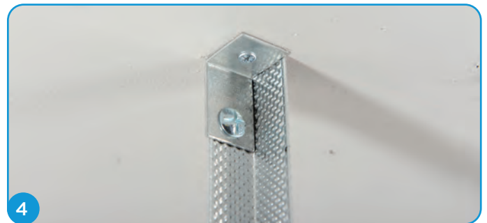
4 Suitably fix these hangers to the soffit at the required centres. For Gyptone BIG™ installation, hangers to be at 1200 mm centres. For Rigitone® Edge installation, hangers to be at 1000 mm centres.
