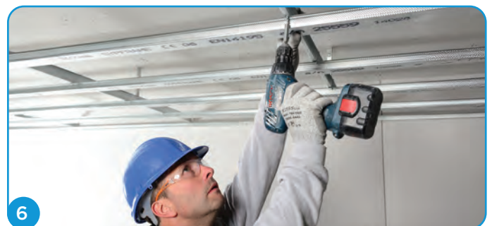
6 Use Gyproc Wafer Head Jack-Point Screws to fix Gyframe MF5 Ceiling Sections to the underside of the Gyframe MF7 Primary support at required centres. For Gyptone BIG™, MF5 Ceiling Sections to be installed at 600 mm nominal centres. For Rigitone® Edge, MF5 Ceiling Sections to be installed at 330 mm nominal centres.
