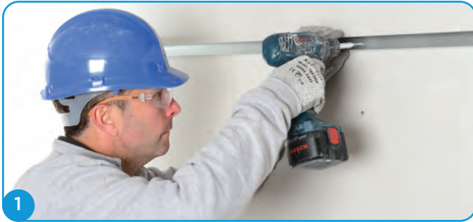
1 Fix Gyframe MF6 Perimeter Channels to the perimeter walls at 600 mm centres.
