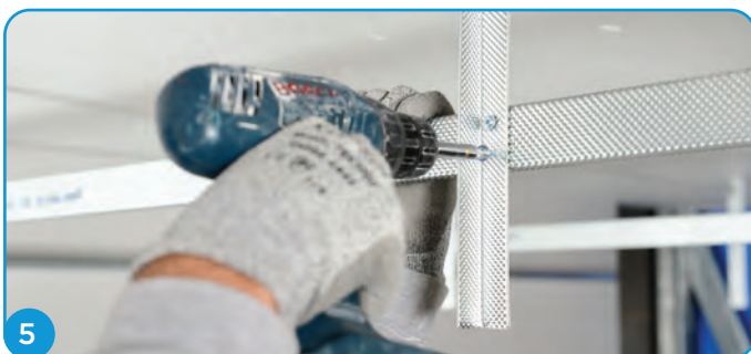
5 Position Gyframe MF7 Primary Support Channels then use Gyproc Wafer Head Jack-Point screws to fix the hangers to the side of these channels. Use two screws per hanger. For Gyptone BIG™, MF7 Primary Support Channels at 1200 mm centres. For Rigitone® Edge, MF7 Primary Support Channels at 1000 mm centres.
