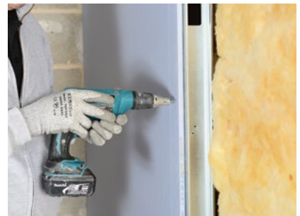
Gyproc plasterboards are then fixed to the Gypframe framework with Gyproc Jack-Point Screws.
