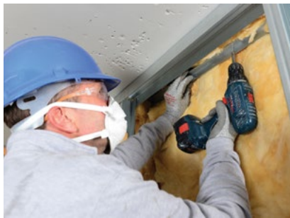
Insulation is added to the partition cavity.
