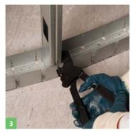
• Locate 70mm Gypframe metal studs into the Gypframe 72 EDCL 80 CurveLiner Channel at required centres. Crimp each stud into the channel at the head and base or fix with Gyproc Wafer Head Jack-Point Screws.
