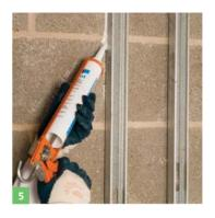
• Apply Gyproc Sealant to both sides of frame perimeter to provide optimum acoustic performance.
