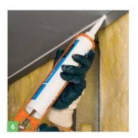
• Apply Gyproc Sealant as a continuous bead to the perimeter of the framing on both sides before boarding commences, to ensure acoustic performance.
