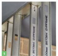
• Fit Gypframe T Studs vertically within the Gypframe Floor & Ceiling Channel at 300mm centres (Gypframe 'C' Studs to abutments – see Junction detail 12). Alternate clips on either side of the Gypframe T Stud to give the staggered stud framework.
