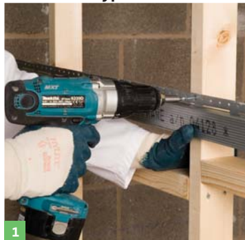
2 Resilient Bar fixed to one side
