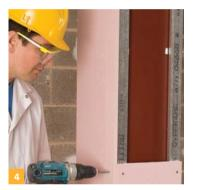
Cut boards to width and fix to all framing members at 300mm centres using Gyproc Drywall Screws. Start with a half length board on opposite sides to stagger board joints around the column.
