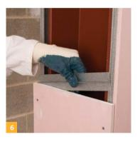
• Fix to vertical channels using Gyproc Wafer Head Drywall Screws, and when board fixing provide an intermediate screw fixing through each board end into the nogging.
