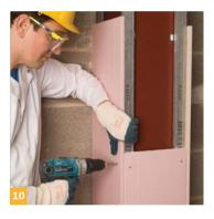
• Cut boards to width and fix to all framing members at 300mm centres using Gyproc Drywall Screws. Start with a half length board on opposite sides to stagger board joints.
