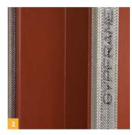
• The Gypframe GL1 Lining Channel stand off from the face of the structural steel frame is 25mm and 10mm from the edge of the flange.
