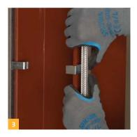
• Snap Gypframe GL1 Lining Channel section over the clips to form the steel framework.
