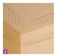
• Scratch plastered or painted areas which will be in contact with the profile to provide a key for the adhesive, and brush away any dust or loose material.
