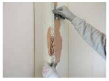
Angle Bead is fixed to the plasterboard angle by embedding in the finish plaster.
