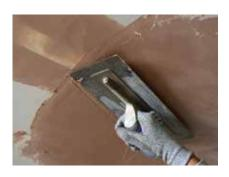
Gyproc plaster is applied with firm pressure, built out to the required thickness in two applications and trowelled to a smooth matt finish. Good site practice should be followed, as outlined in BS EN13914 - 2: Design Considerations and Essential Principles for Internal Plastering.
