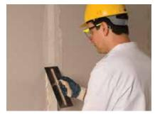
Where there is an increased risk of cracking, or where joints exceed 3mm, the joints are reinforced with Gyproc Paper Joint Tape\* bedded in Gyproc plaster.
