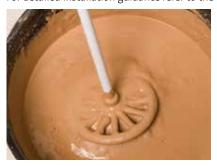
Gyproc plasters should be mixed by adding to clean water and using clean mixing equipment. Contamination from previous mixes must be avoided as this can adversely affect the setting time and strength.
