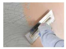
Once the Gyproc undercoat plaster has set, Gyproc Finish Plaster is applied with firm pressure, built out to the required thickness in two applications and trowelled to a smooth matt finish. In some circumstances it may be necessary to control the suction with Gyproc GypPrime. Good site practice should be followed, as outlined in BS EN 13914 - 2 Design considerations and essential principles for internal plastering.
