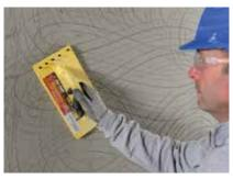
The final coat is ruled to an even surface and lightly scratched to form a key for Gyproc Finish Plasters.
